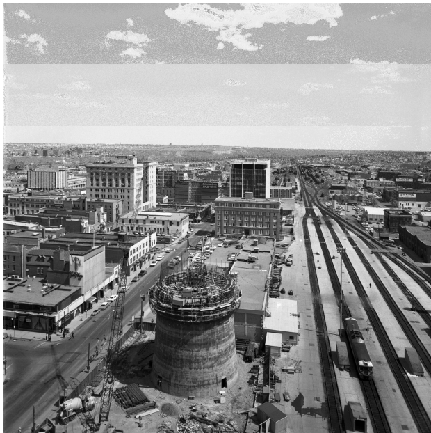
Photo 3. Construction of the Husky Tower in 1967 (Glenbow Archives)
